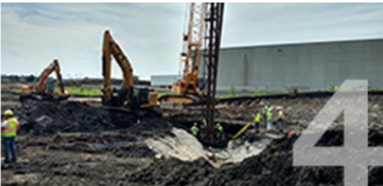
Driving test piles for the timber pile foundation of the North Box Culvert before the area is excavated.
