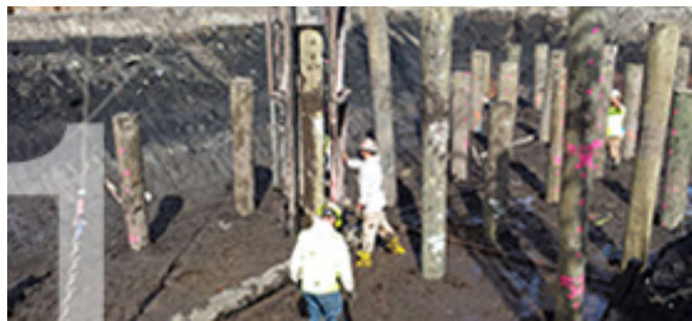
Timber pile driving for the foundation of the North Box Culvert as part of the Advance Earthwork of IL 390 & I-490 Interchange
