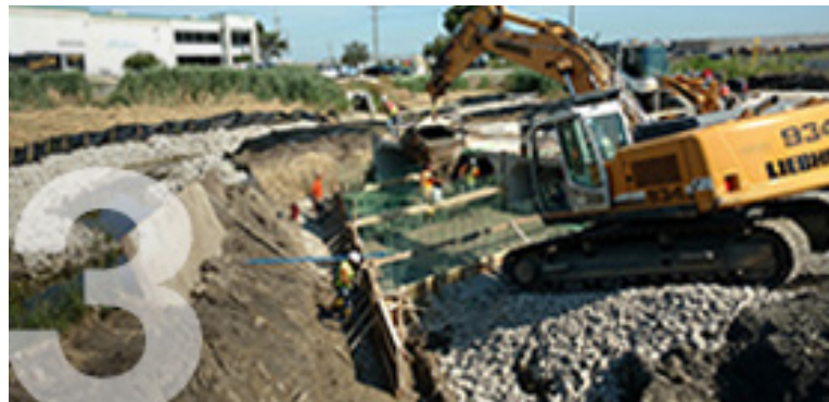
Forming for the head wall at the south end of the South Box Culvert (for Willow Creek relocation).
