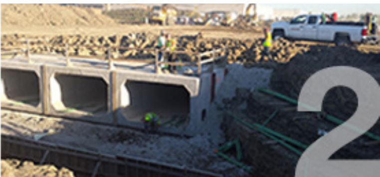
South Box Culvert installation under South Frontage Road along IL 390.
